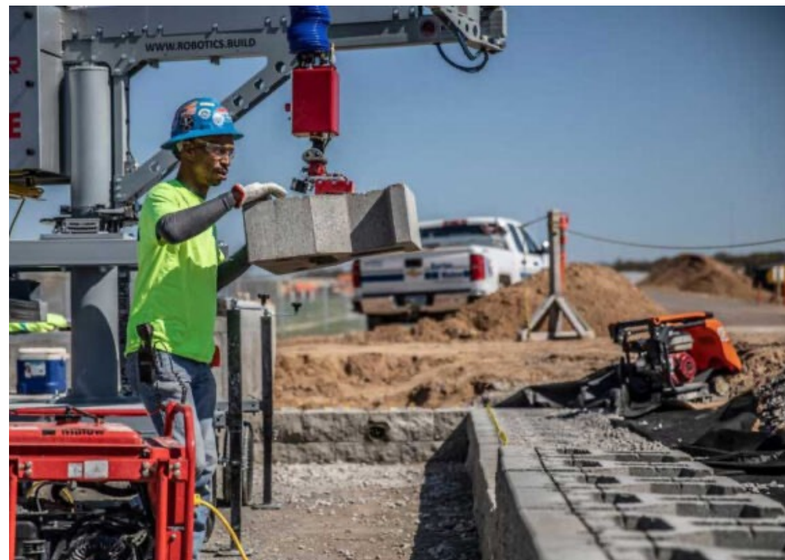
The construction firm Barton Malow already uses simple robots on some job sites, such as this MULE, which helps workers place retaining wall block. (Photo courtesy Construction Robotics)
